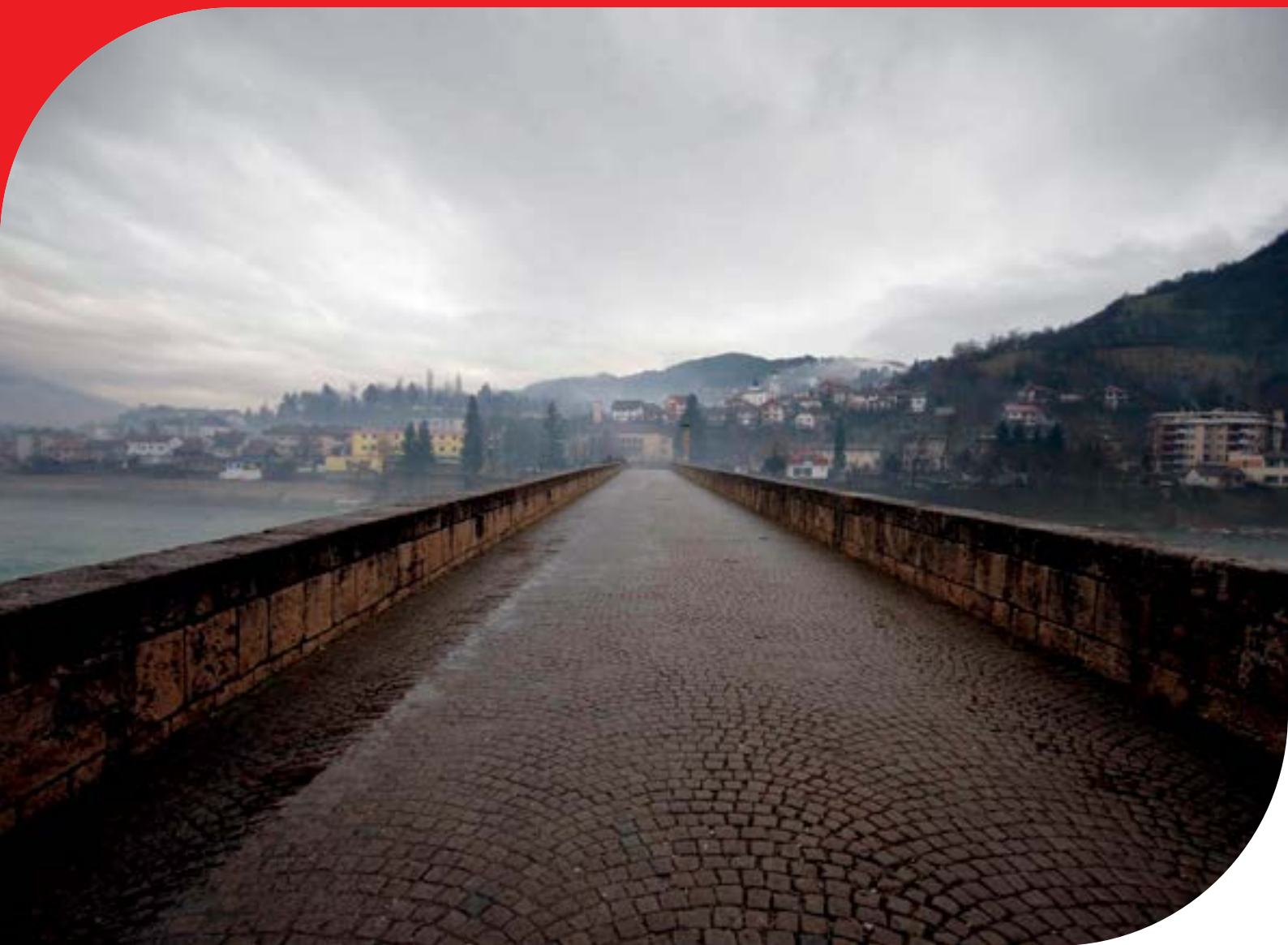
Višegrad Bridge: Bosnia and Herzegovina
